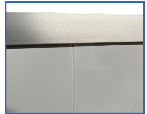
Close Up View of Butt Seam
